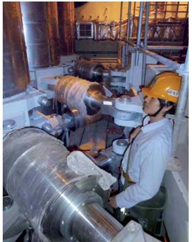
Commissioning of type 30
