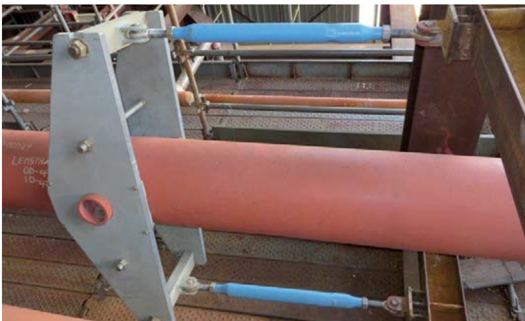
Horizontal axial stop with rigid strut type 39 and pipe clamp type 34 incl. spacer
