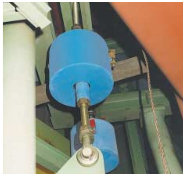
Spring hanger type 22 with clevis mounted.
